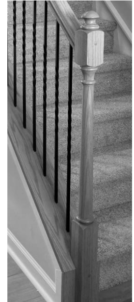
Spindles & Newell Post per plan Stair Railings
